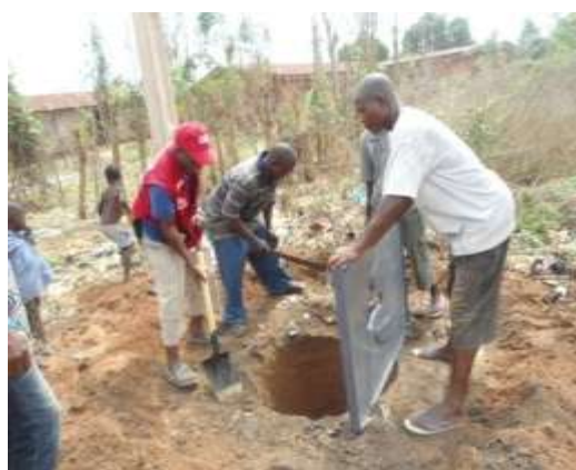
Construction of emergency latrine
